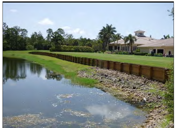
Wooden Timber Bulkhead, Driving Range
