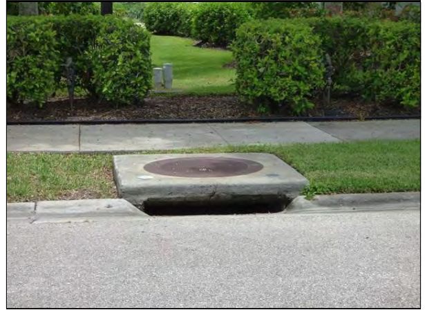
Stormwater Drainage Curb Inlet
