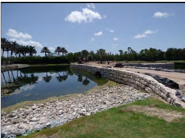
Rock Wall Bridge and Culvert, Hole 4
